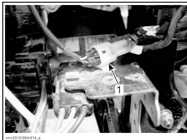
1. Connector of auxiliary line pressure transducer
